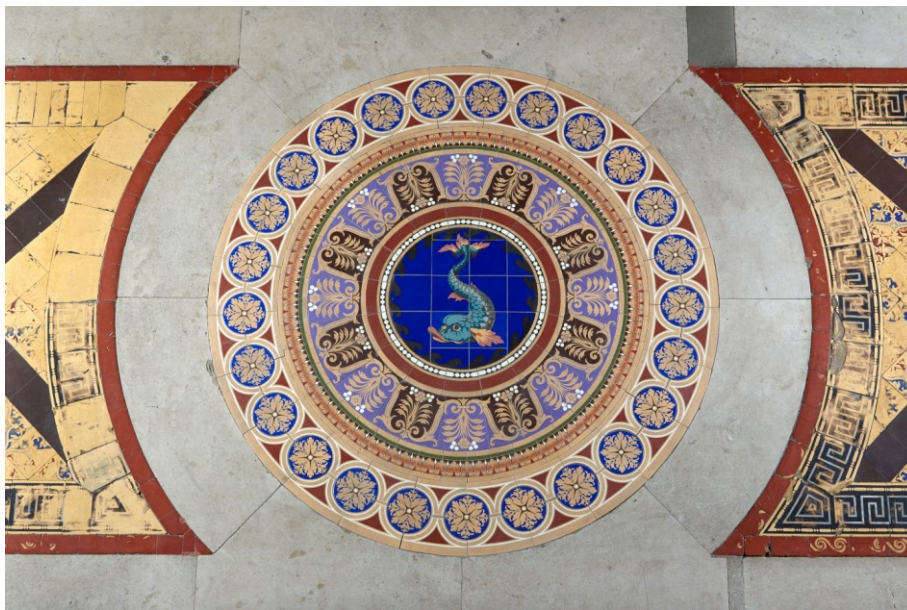
Restored roundel at St. George's hall
