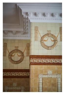
reveals. This running border also involved the hand-manufacture of bulb-glazed, square tiles in two colours, accurately matched in hue. Rising towards the ceiling is a band of plain yellow tiles for which Jackfield manufactured some 1200 replacements.
